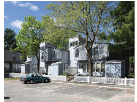
SPRINGFIELD APARTMENTS Springfield, MA
